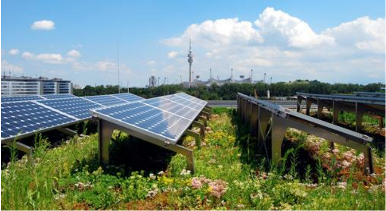
Greenscape green roofs with solar panels
