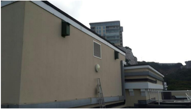
Starling boxes installed by the Department of the Environment and Climate Change at the Dementia Care Centre.
